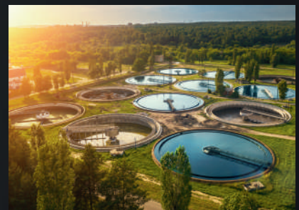
Sewage treatment plants
